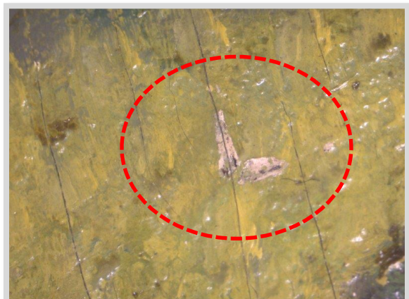
10. Micrograph image (x6.4 magnification) detailing a site of paint loss (circled in red) on the lower, left side segment of the grass embankment.
